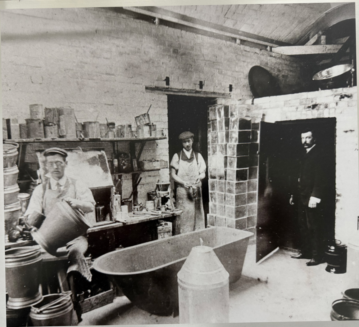
1904 - Japanning Shop at 45 Colombo Street W.H. Harris on right
